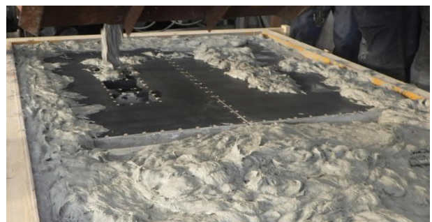
Photo.2 Pouring HPFRCC on power transfer coils
