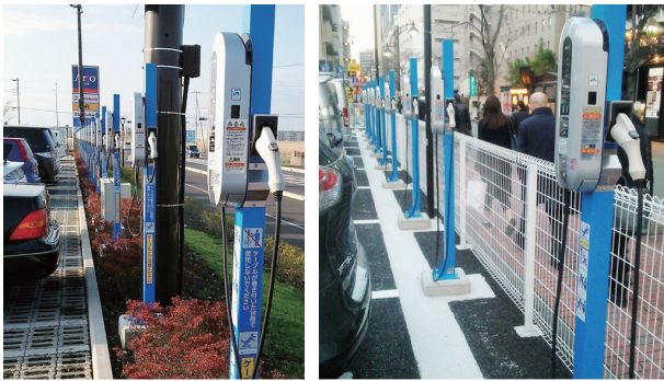
Fig. 5 Examples of Large-scale Normal Charger Installations (Left: Suburban large-scale commercial facility, Right: Metered parking lot).
